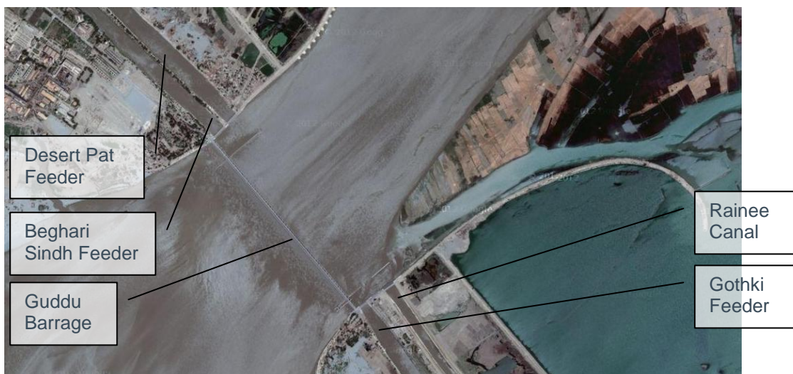
Figure 22. Aerial view of Guddu Barrage and off-taking canals.
