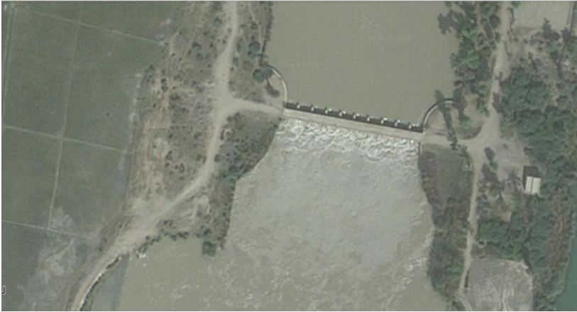
Figure 16. Aerial photograph of Rohri RD15 fall regulator
