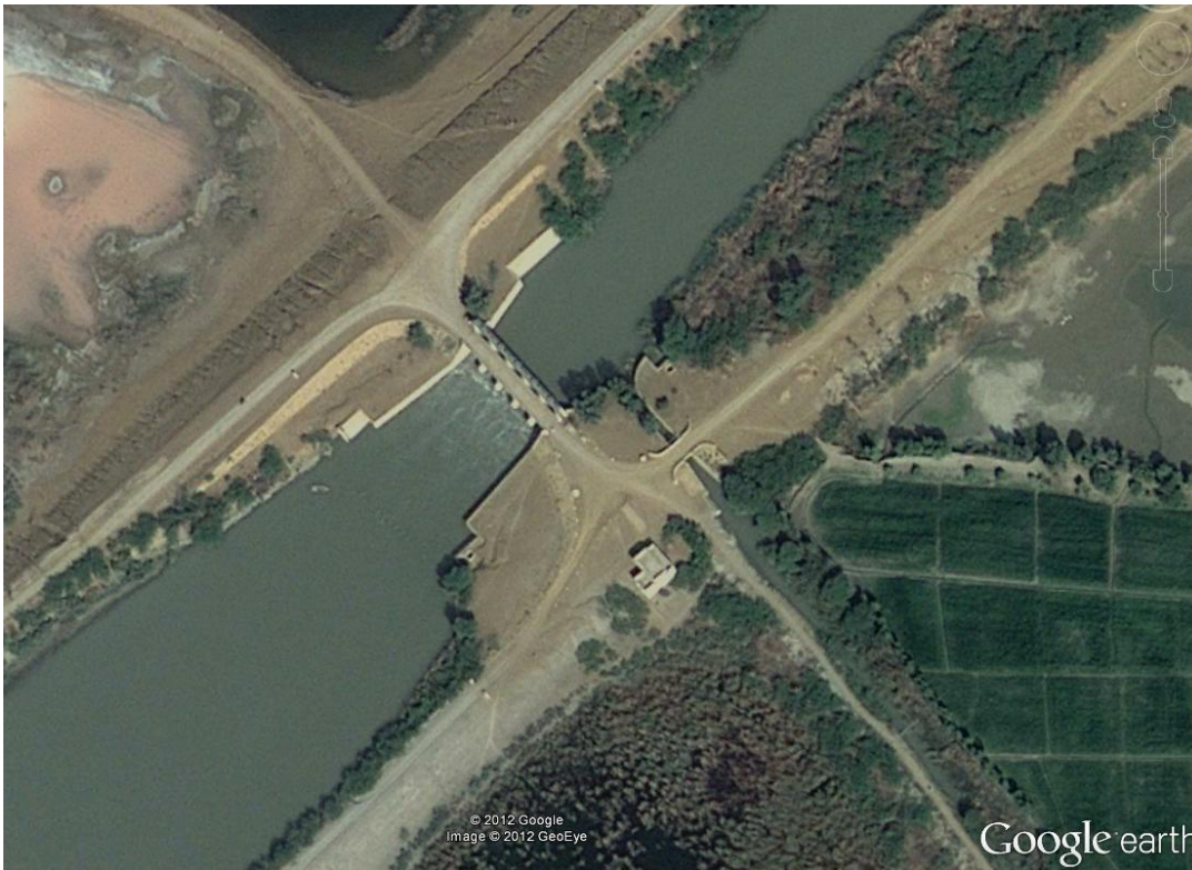
Figure 28. View showing immediate vicinity of KB link canal, RD 19.5.
