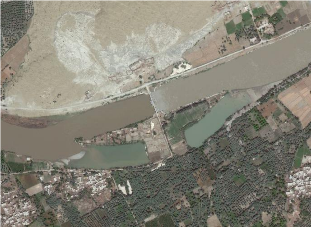
Figure 32. Structure RD 26 on the Nara Canal, with previous diversion channel showing.
